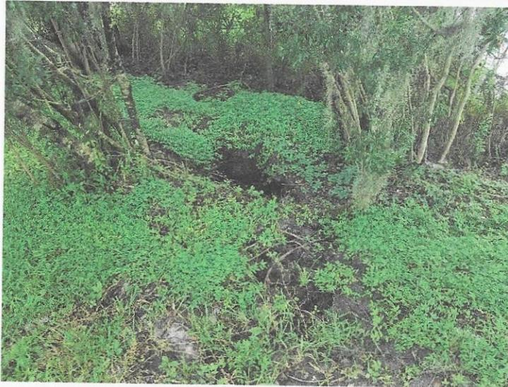
ABM is going to remove the undergrowth and fill the hole first with rock, then gravel and finally dirt. Mike (City) agreed that if this were to reoccur, he would bring in equipment to try and visualize the stormwater conveyance to make certain that it is not involved.
