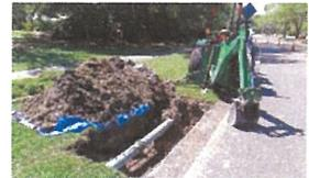
Complicating the repairs is the fact that often these lines run on top of the City's potable water system, and are adjacent to communications cables.
